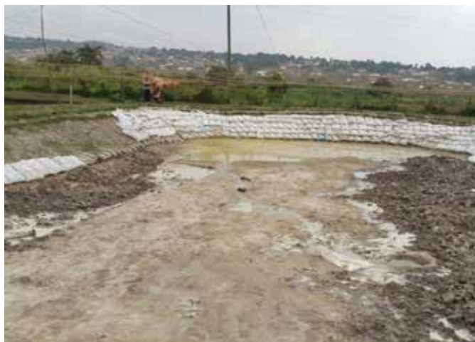
Proper construction techniques are a common challenge for farmers. Proper pond siting and construction safeguards against water seepage and would prevent the need to use sand bags to hold walls and prevent seepage.
